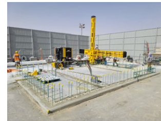
Application of 3D Printer (HUGRS project in Saudi Arabia)
