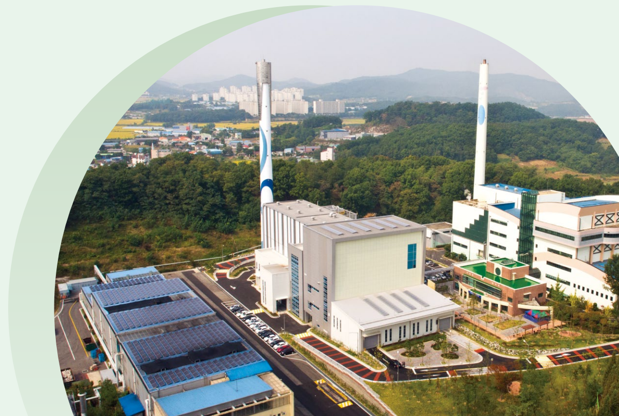
Incineration Plant in Cheonan
