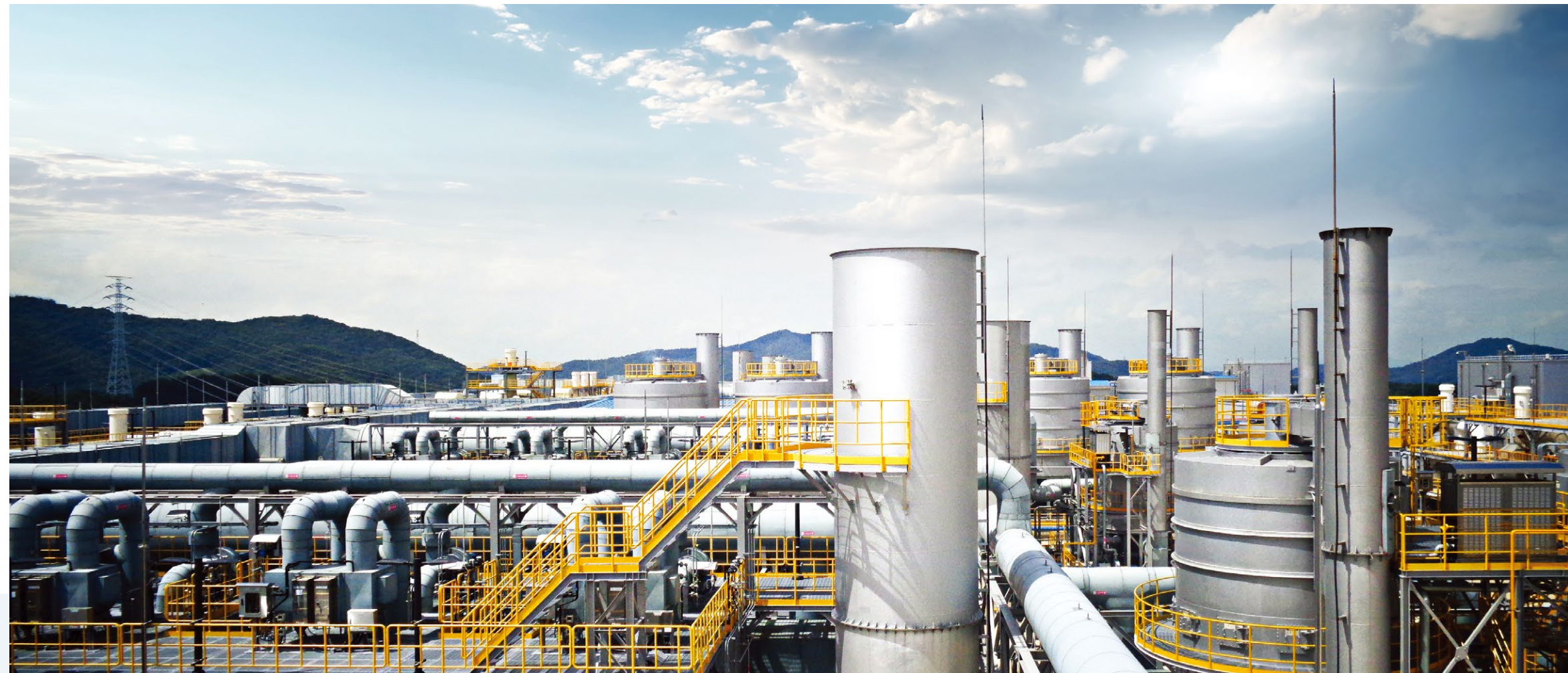
Samsung Display Asan Air Pollution Prevention Facility Project
